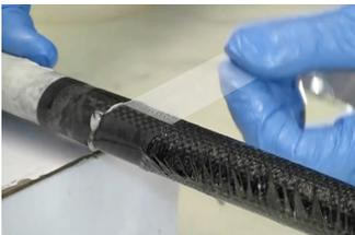
The next step is to apply the heat shrink tape over the repair in a spiral pattern.
